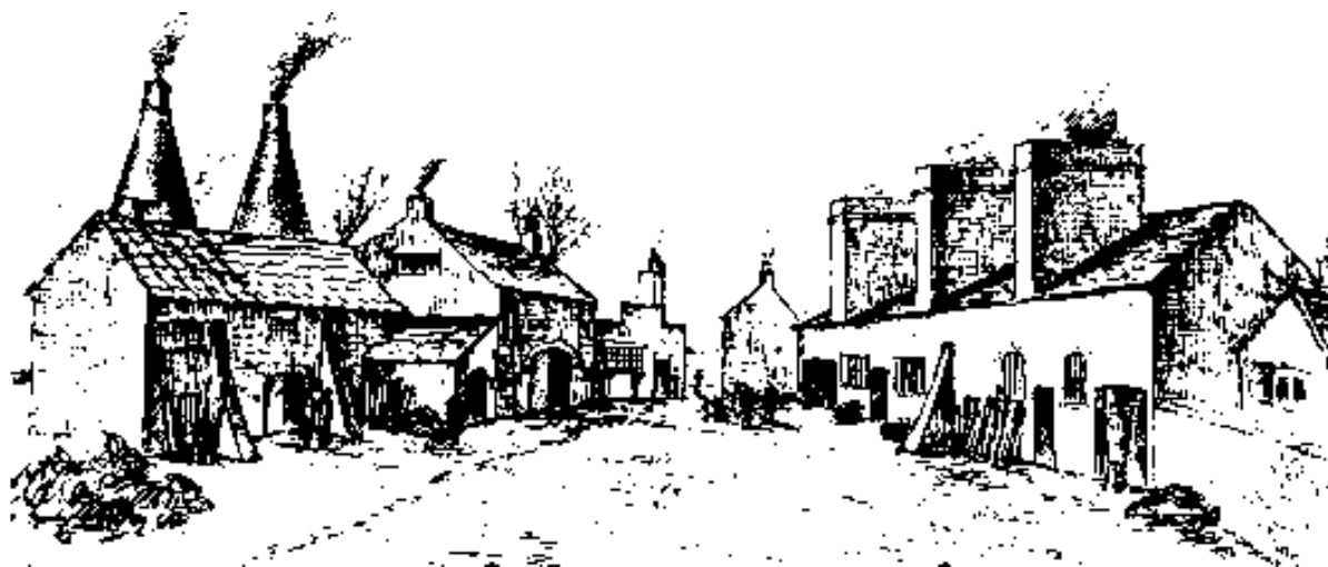
Figure 14.5: Stone and Brickwork buildings at Huntsman's Attercliffe Works, circa 1787
